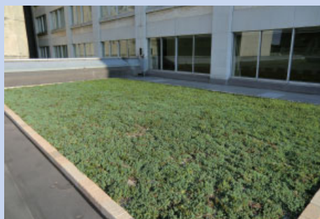
Establishment of rooftop garden systems
