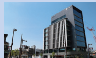
The Ichibanmachi Square Building
