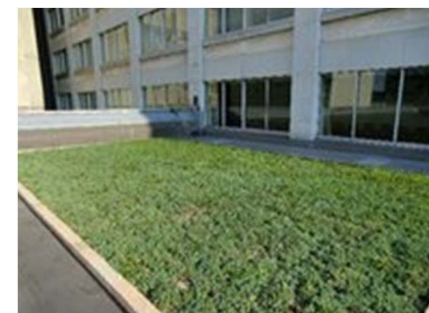
Greened rooftop at headquarter of Hokuriku Bank
