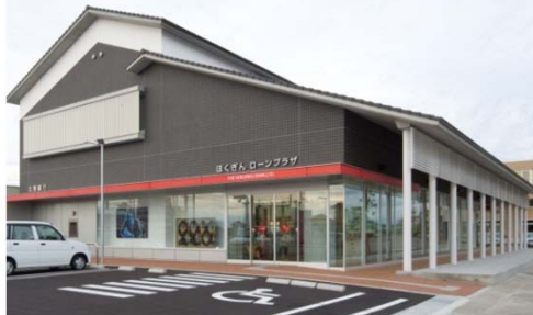
Kanazawa Tonya-machi Branch (Hokuriku bank) (Relocated and newly opened in Oct. 2010, with solar power equipment on the roof and LED signboard in front)
